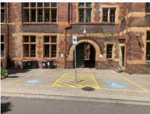
North entrance with ramp and lift access on Manning Road along with disability parking in front.
